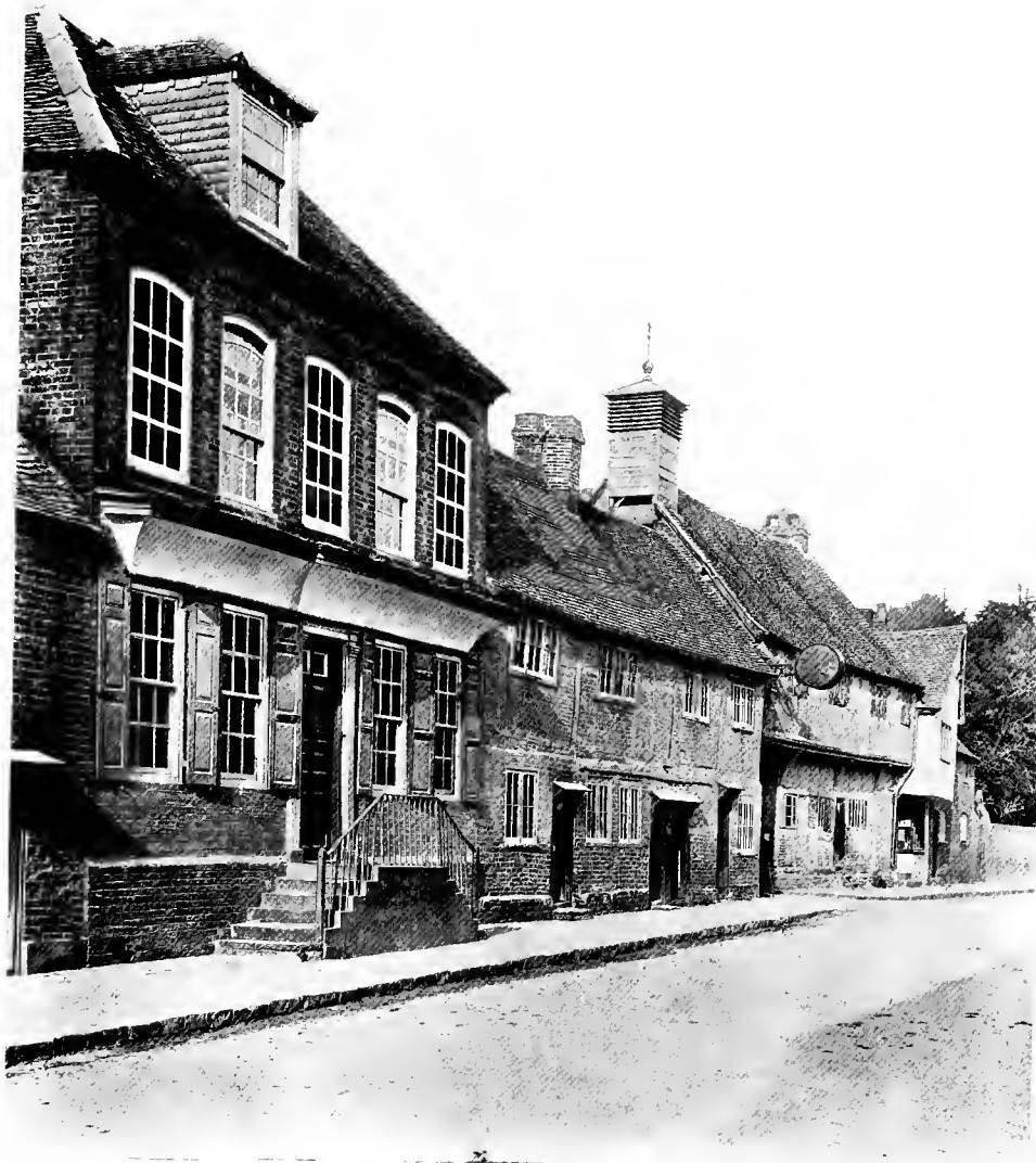
STREET AT WEST WYCOMBE, BUCKS
